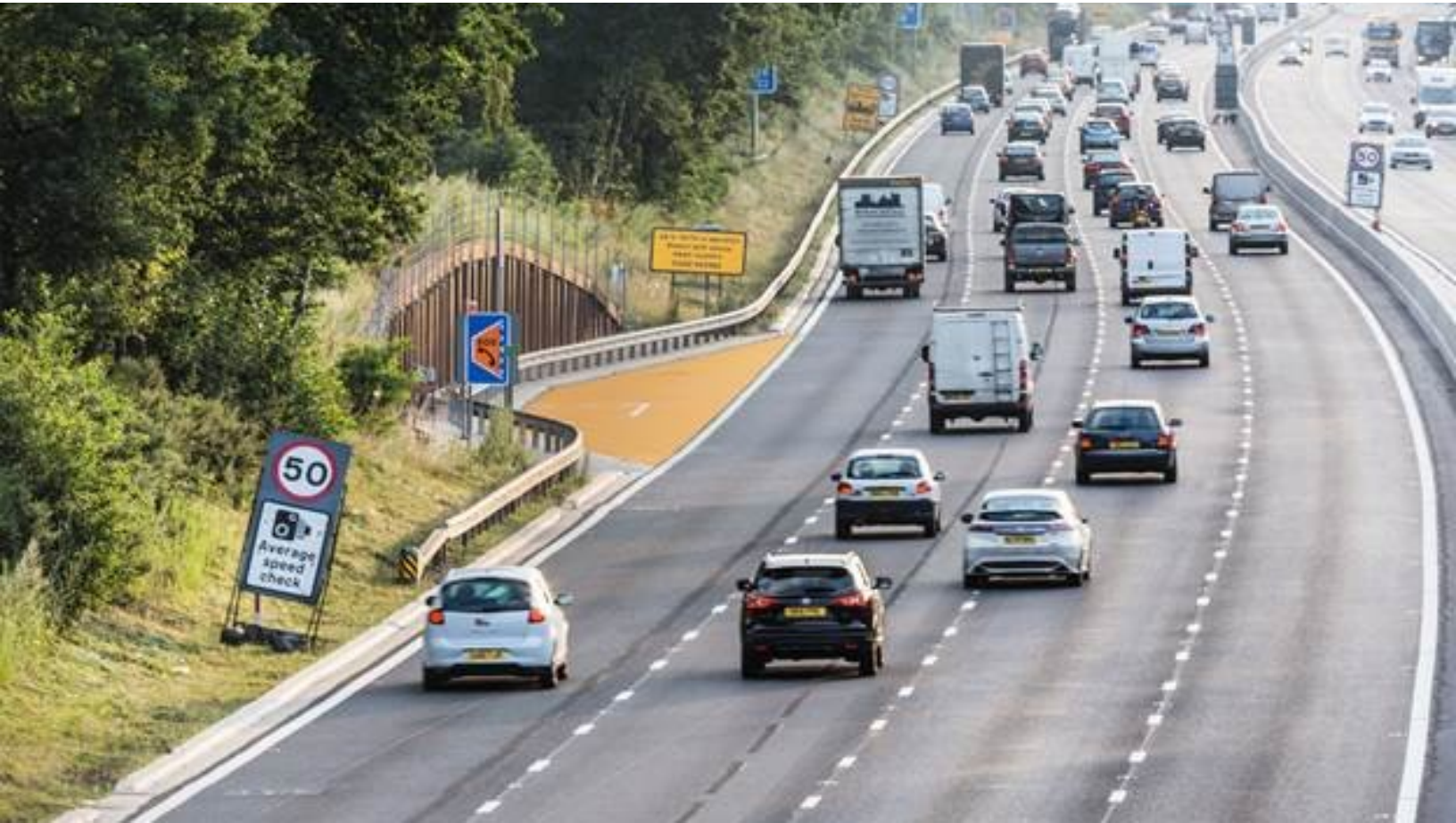
Improved visibility - the bright orange SOS-signed emergency refuge area on the M3 near Camberley
